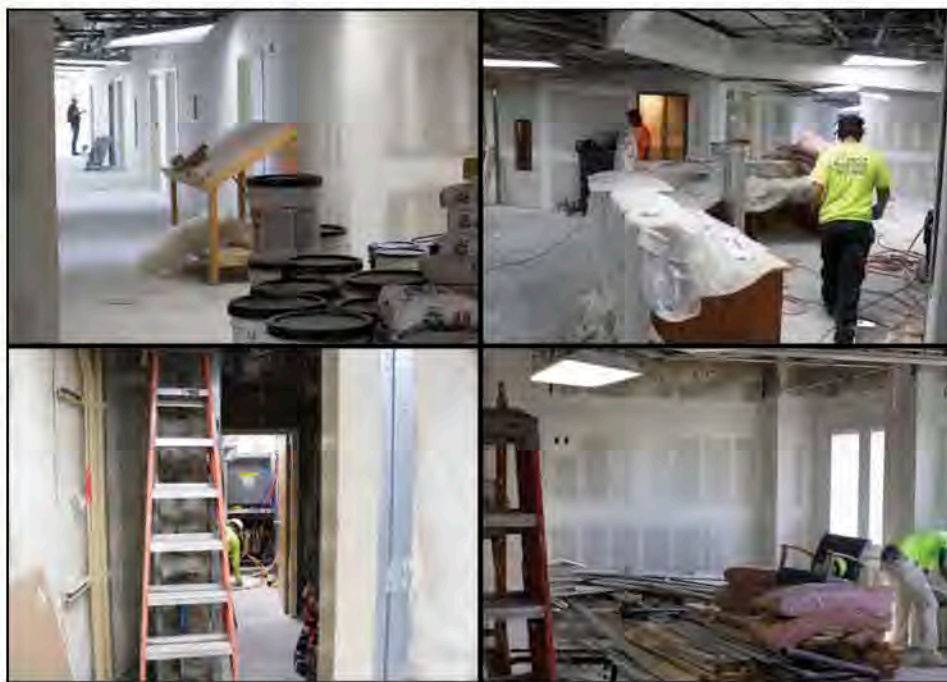
Above: View of Construction site of what will be the Behavioral Health Unit at Lehigh Regional Medical
